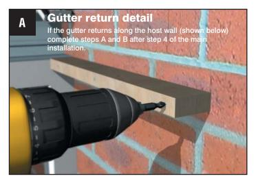
Ensure the treated timber baton (49mm x 20mm) is level, then fix into position.
