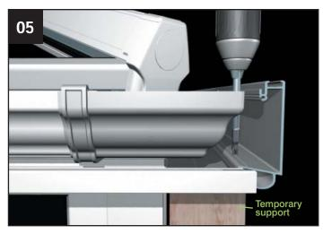
Offer up the middle Cornice section into position, (it may be advisable to temporarily support the lower Cornice section whilst fixing) secure using fixings provided (CRN007). (Long reach driver required).
