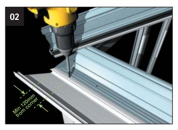
Remove the under gutter trim and dispose of it. Prior to fitting gutter offer up the lower Cornice section then secure into position using the fixings provided (CRN007). **Please note: Always start with the front facet!**
