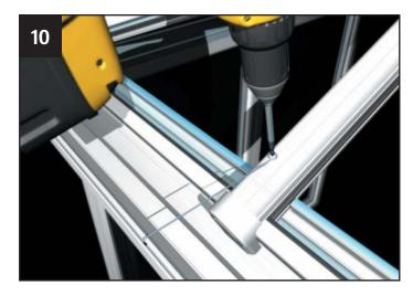
Secure the upper Cornice section using the wire ties at each glazing bar. Hook the wire tie into the pre-drilled hole in the upper Cornice section and screw fix into the glazing bar, ensuring the upper section remains parallel to the frames/roof line.
