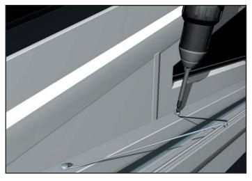
Fix wire ties at an angle as shown, ensure the Cornice is parallel to the frames/roof line.
